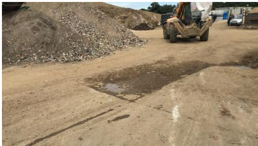
The telehandler involved in the accident | Image: HSE
