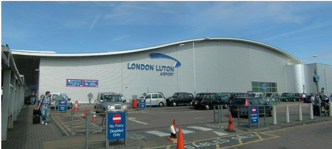
The exterior of London Luton Airport (Wikipedia commons)
