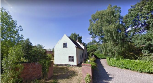
The house on Field Lane before renovation – including the gates
